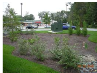
This is an example of a bio-retention facility, located at the Rt. 10 Sonic.
