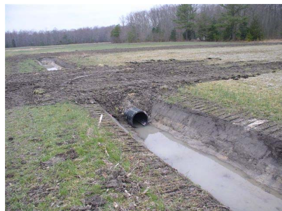
Newly installed crossing pipe in a recently cleaned-out tax ditch.
