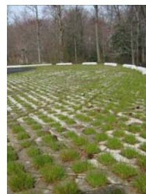
Porous pavers used for extra parking or travel lanes allow for water to infiltrate into the ground and cause less stormwater runoff.
