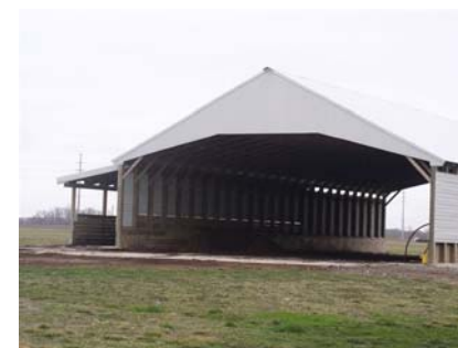
Poultry manure storage structures with attached channel composter.
