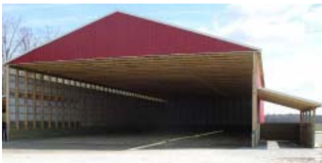
Poultry Manure Storage Structure with Lean-to Channel Composter
