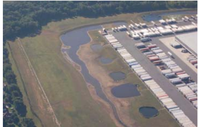
Stormwater Management Ponds
